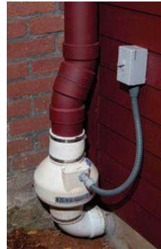
*Per EPA guidelines, the radon exhaust fan is installed outside the building and is connected to the suction point in the basement with PVC pipe.*
