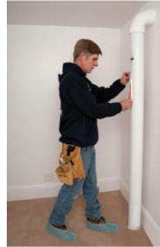
*Indoor piping of a radon system is usually installed in a basement utility room or an unfinished corner of the house.*
